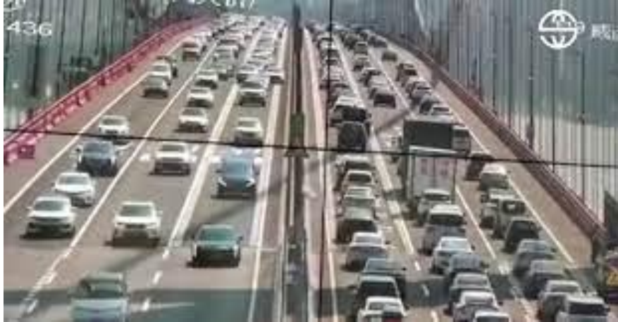
Heavy traffic, complex large bridge
