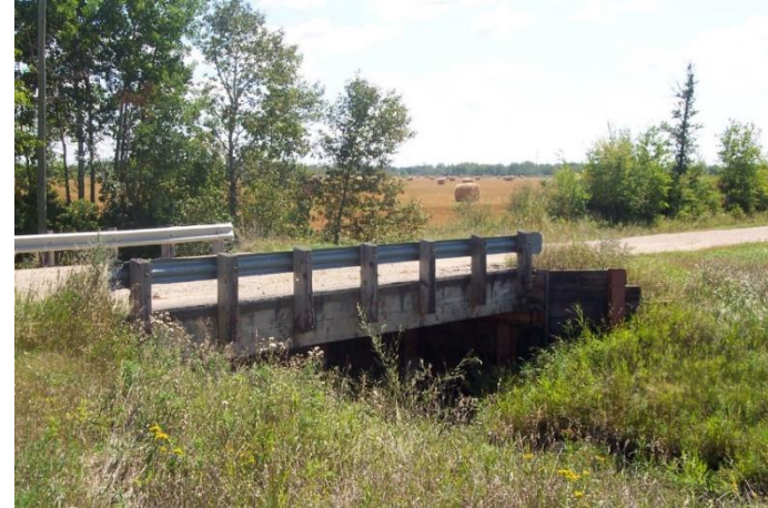
Low traffic, simple small bridge
